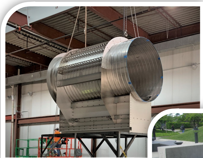
Figure 1 - Customer Installation of GA fabricated parts
